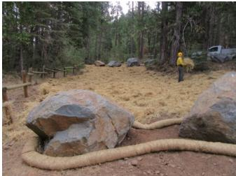
Volunteers installed straw wattles, scattered hay, and repaired wooden fence posts to deter illegal use by OHVs of areas along Deer Creek. The wattles and hay reduce the movement of sediment into the adjacent stream (see pictures to the left taken during and after volunteers spread the hay and installed the straw wattles on a bare, eroding hillside).
