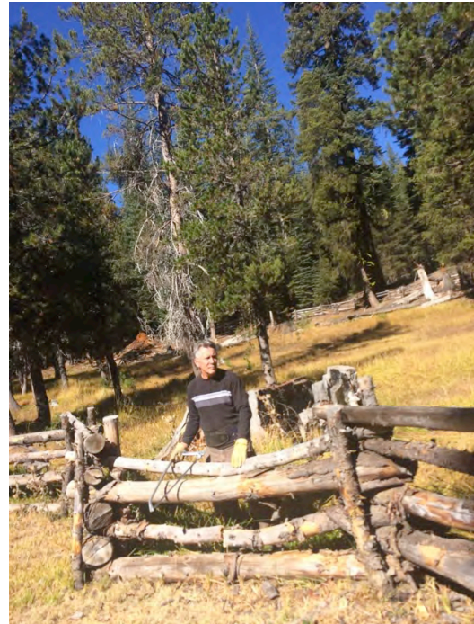
In 2016, the fence that took so many projects to build is holding up well, but a few logs needed reinforcement or replacement.
